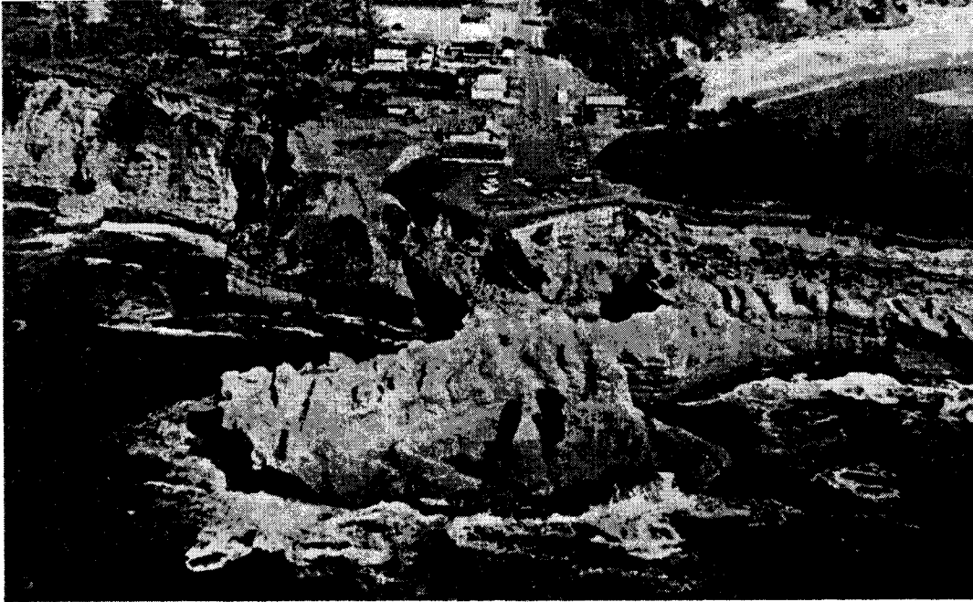
Photo 57. Devils Punch Bowl State Park at Otter Rock, a marine terrace on a sandstone headland. Wave erosion removes terrace sediments faster than the sandstone, continually reducing the margins of the park area.
