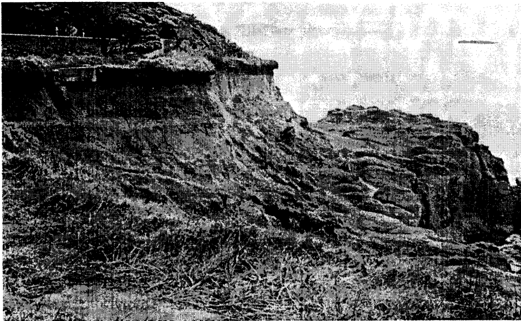
Photo 58. Close-up of Devils Punch Bowl area. Erosion has removed former stairway access to the Punch Bowl on right. Remains of old walkway projects from cliff at left.
