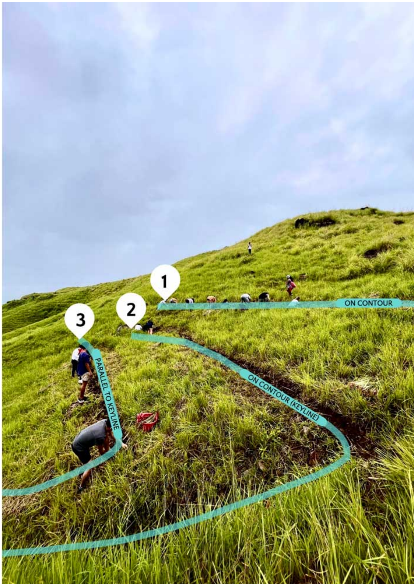
Planting vetiver grass hedgerows on keyline geometry to halt erosion and sedimentation
