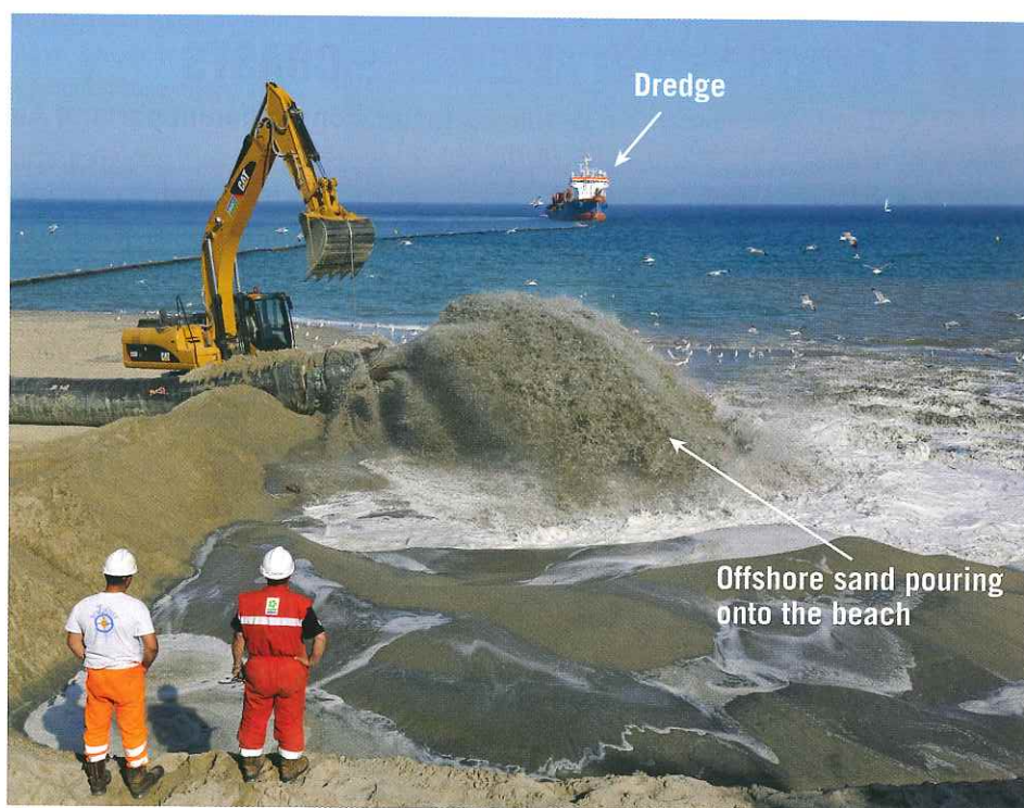
FIGURE 15.28 Beach Nourishment If you visit a beach along the Atlantic coast, it is more and more likely that you will walk into the surf zone atop an artificial beach. In this image, an offshore dredge is pumping sand to a beach. (Photo by Michael Weber/Alamy)
