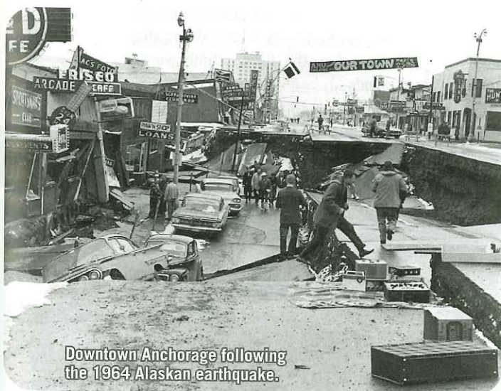
FIGURE 8.20 Ground Failure Caused This Street in Anchorage, Alaska, to Collapse (Photo by USGS)
