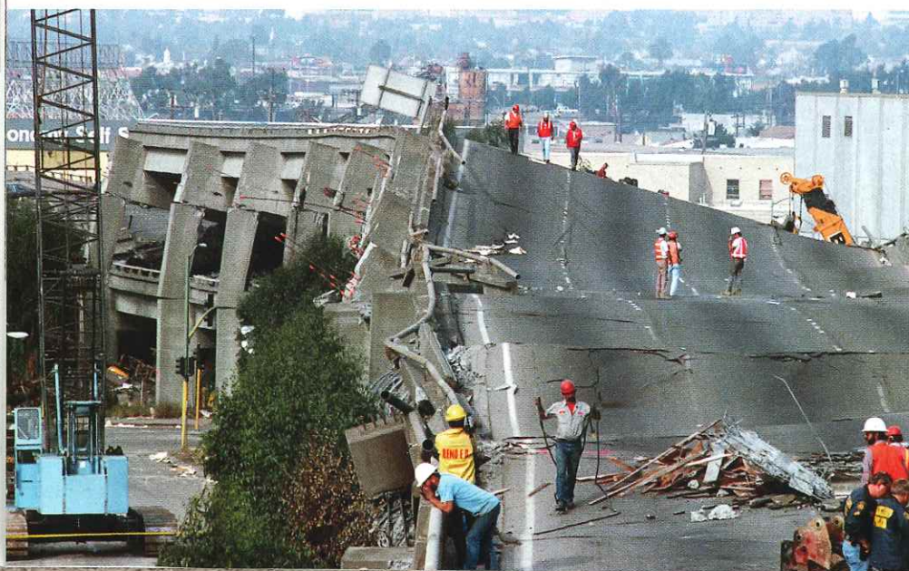
FIGURE 8.30 Collapse of the Double-decked Section of I-880 This section of a double-decked highway, known as the Cypress Viaduct, collapsed during the 1989 Loma Prieta earthquake. (Photo by Paul Sakuma/AP Photo)
