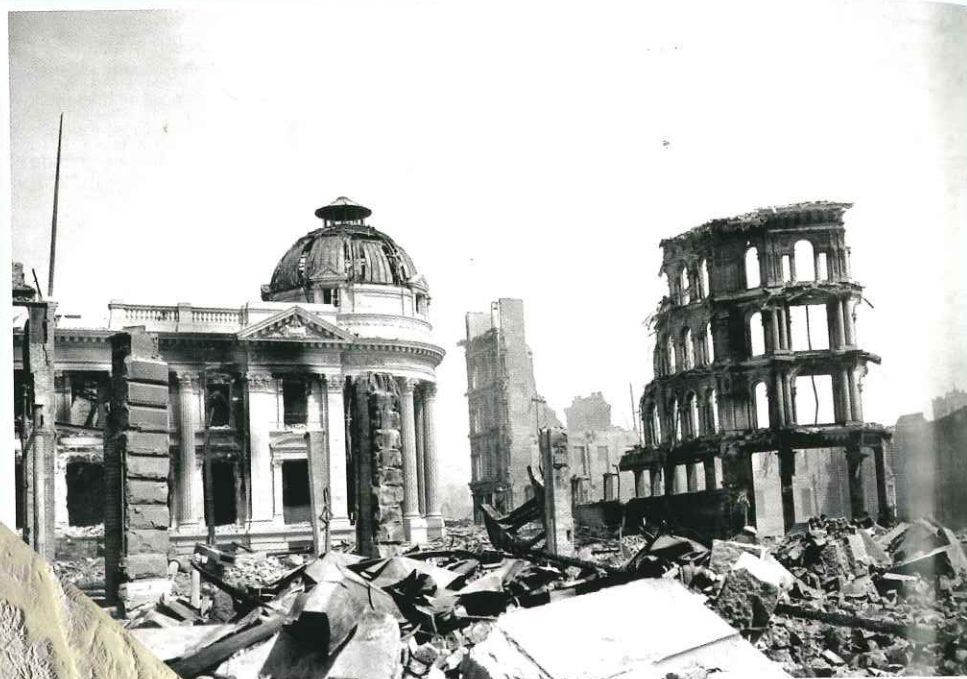
The 1906 San Francisco earthquake was the most devastating in California's history. The quake and resulting fires caused an estimated 3000 deaths and extensively damaged buildings throughout the city. The business district was devastated largely because it was built on land made by filling in a cove. (USGS)
