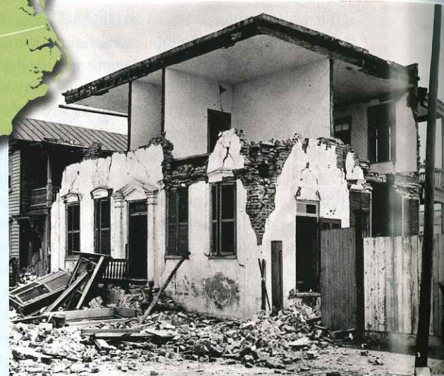
Residence damaged during the 1886 Charleston, South Carolina, earthquake. (USGS)
