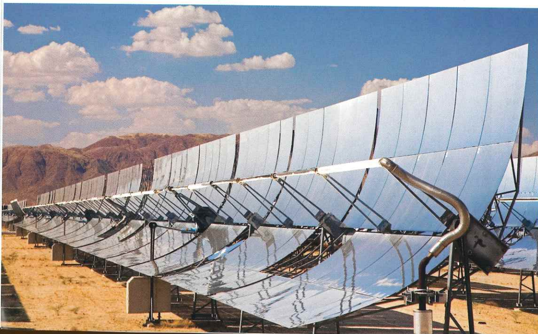
FIGURE 2.33 Solar Energy Is Renewable These solar collectors focus sunlight onto collection pipes filled with a fluid. The heat is used to make steam that drives turbines used to generate electricity. (Photo by Jim West/Alamy)
