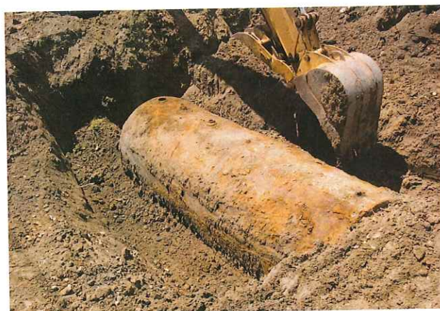
FIGURE 5.38 Potential Sources of Groundwater Contamination Sometimes leaking gasoline storage tanks and materials leached from landfills contaminate aquifers. (Storage tank photo by Earth Gallery Environment/Alamy; landfill photo by Picsfive/Shutterstock)
