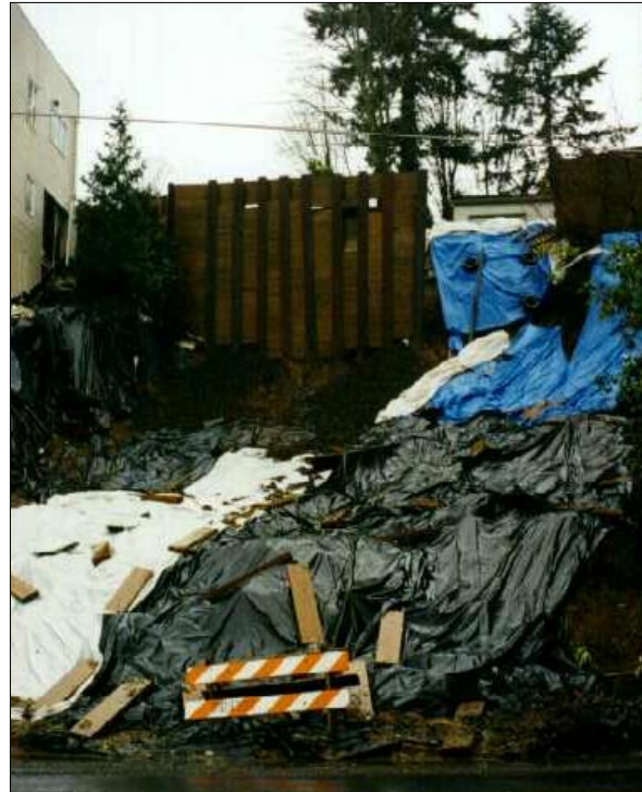
Landslides are a common problem throughout Oregon. This 1996 landslide in Portland's West Hills directly affected at least four lots and two roads. The major damage occurred to the house located across the street from the slide.
